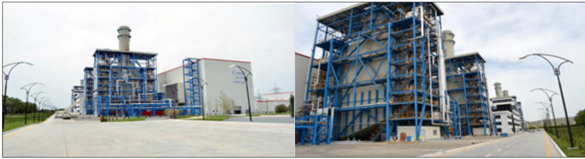
Fig. 1. The new “Janub” Power Plant
